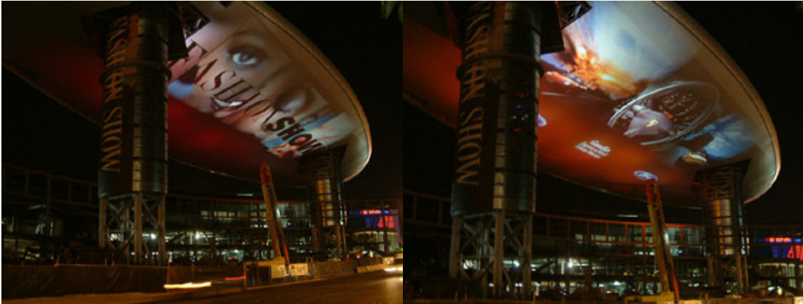
Figure 8. Cloud after cladding installation
