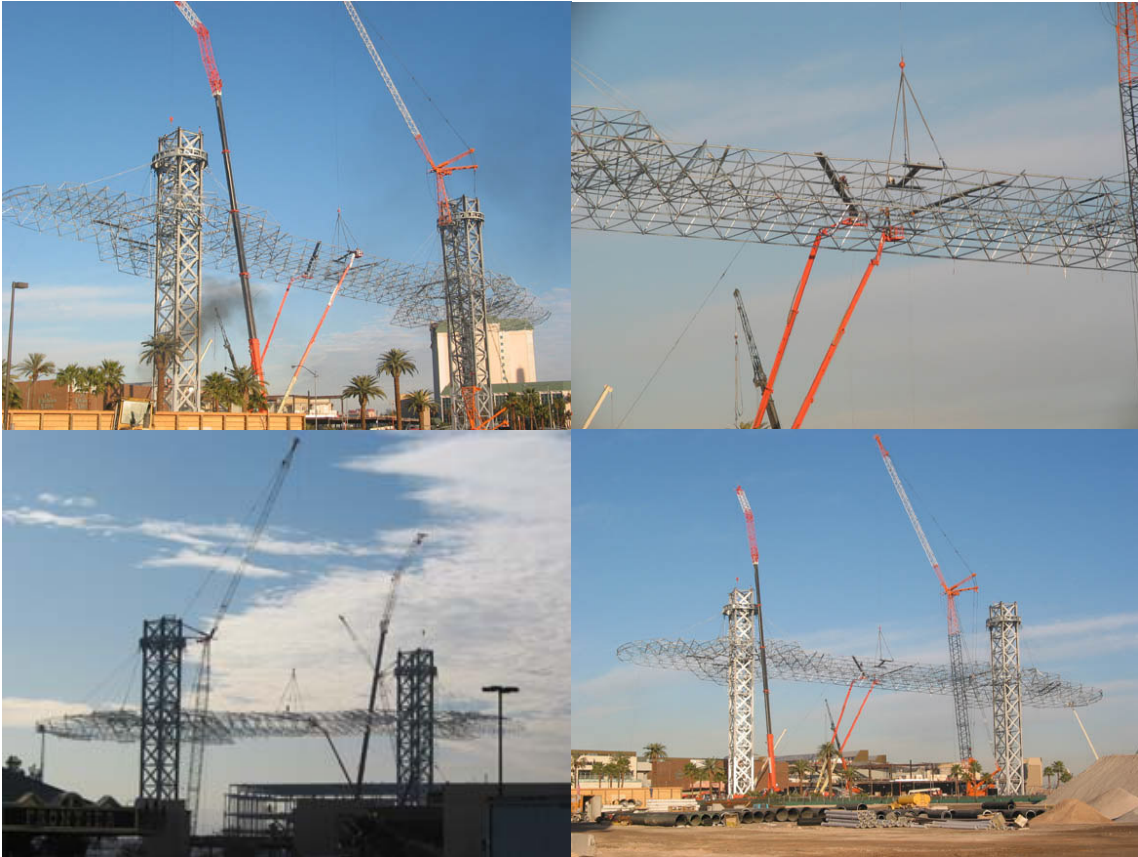
Figure 6. Connecting the north and south segments
