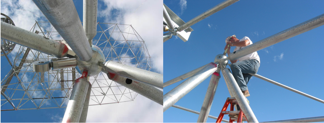
Figure 4. Node Assembly
